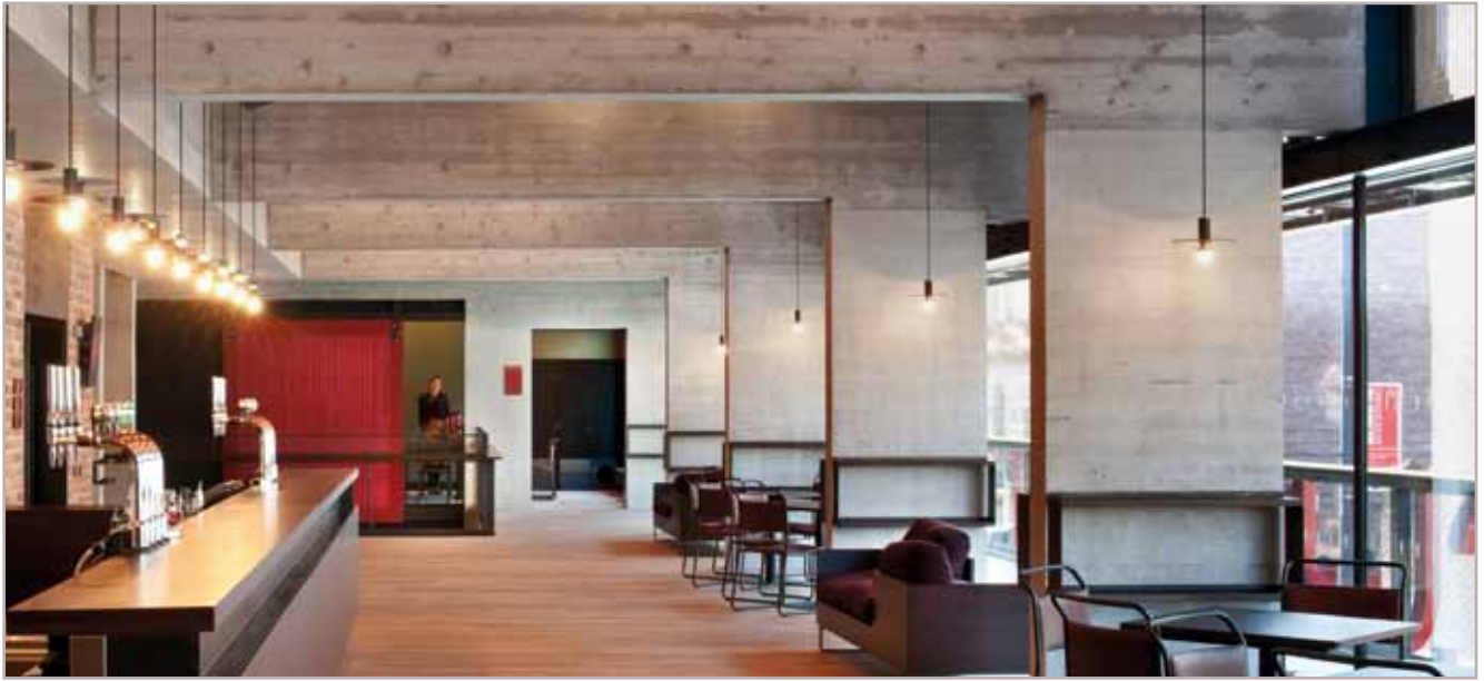
Winner of the 2014 RIBA Stirling Prize, Everyman Theatre, Liverpool uses exposed concrete to provide thermal mass and to pre-cool the incoming air. Courtesy of Philip Vile.
