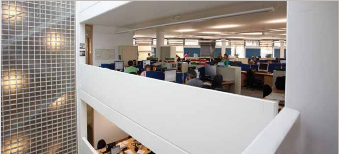
CAFOD Headquarters, Southwark. This building features internal concrete slab soffits which are exposed to provide thermal mass heating and cooling. Photo courtesy of Black Architecture.
